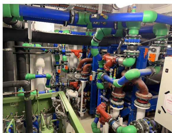
Chilled water system (airconditioning)
